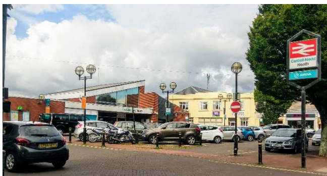
Neath Transport Hub
